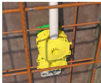
Latch the rear part with conduit onto the front part, then pour concrete.
