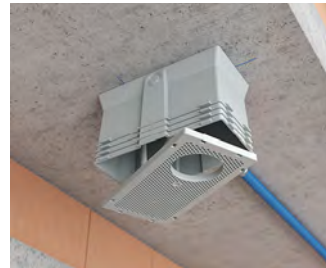
Depending on the required installation diameter ceiling exit of Ø 68 mm or up to Ø 86 mm, turn the front part by 180° and latch into position.
