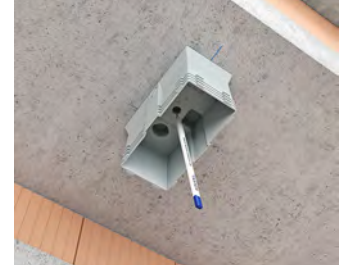
Alternative: Position the installation housing with the alignment markings for the luminaire and mark the drill hole.
