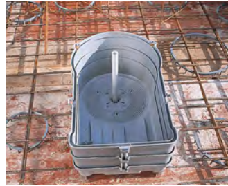
Attach the housing with 2 intermediate frames and a support conduit to the formwork.
