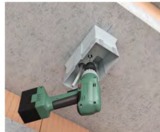
Screw installation housing to the ceiling.
