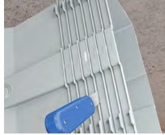
Adapt installation housing to the insulation thickness.
