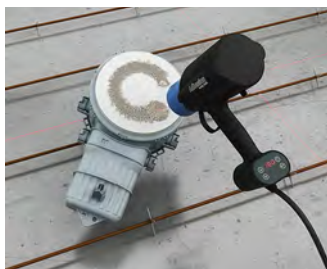
Mounting of the single-piece housing with mineral fibreboard...
