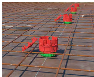
The conduit entries are above the bottom layer of reinforcement – no need to cut the reinforcement bars.
