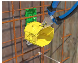
Open the conduit entry.
