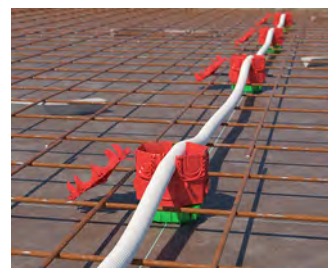
The advantage of the new cable entry is that inserting empty conduits for multiple ceiling junction boxes in one line can take place by simple laying of the installation conduit without cutting it before.
