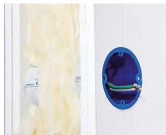
Use of an opposing sound insulation box.
