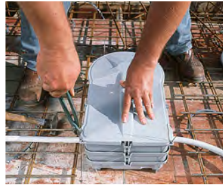
Also secure the housing to the reinforcement.
