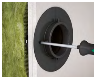
Fix sealing cylinder by tightening the screws (same procedure as with cavity wall boxes).
