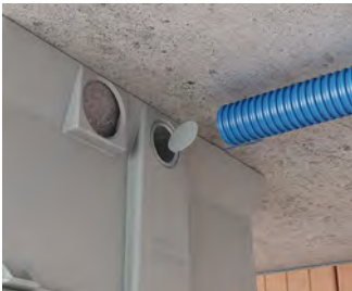
Insert the conduit or cable into the installation housing; fit sealing plug to the conduit.
