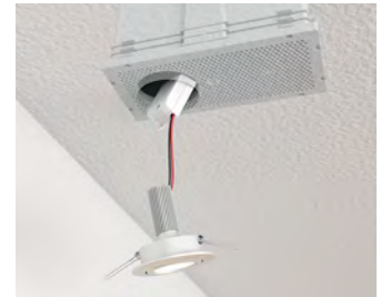
Applying insulation and plaster. Fitting the LED installation spotlight with plenty of space for the ballast device.
