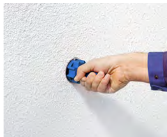
Use KAISER tool Styro55 for fast, easy fitting of the swivels.
