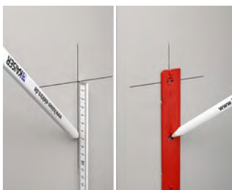
Mark the centre of the upper installation opening in accordance with DIN 18015-3 and the centre of the other installation openings with 71 mm spacing.
